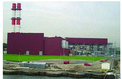
Astoria power plant, New-York, U.S.A.
