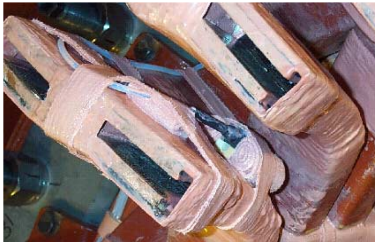
Figure 6: FOA Installation on End-winding
