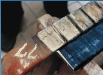
Abrasion of a bar insulation from in-slot vibration (radial) against stator lamination compared to a new bar.
