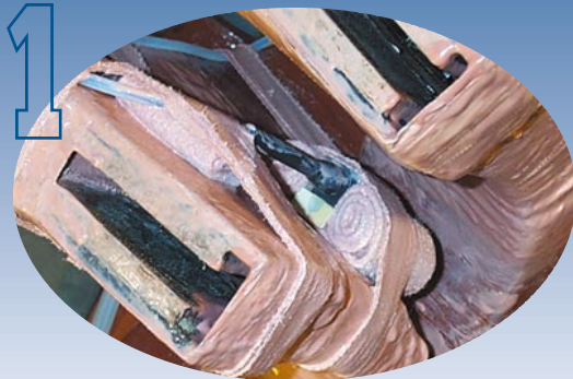
FOA INSTALLATION ON END-WINDINGS OF TURBOGENERATOR
